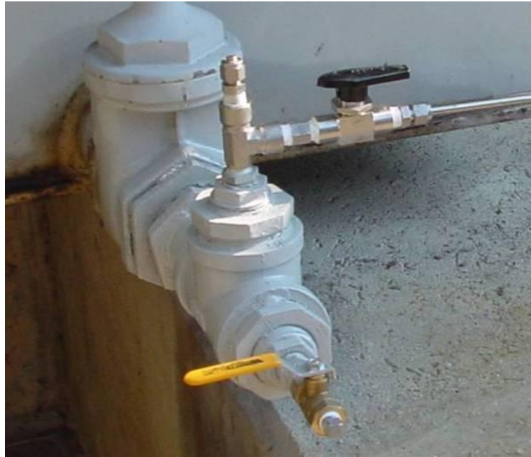
Figure 12: Bleed assembly on threaded-type oil return valve
